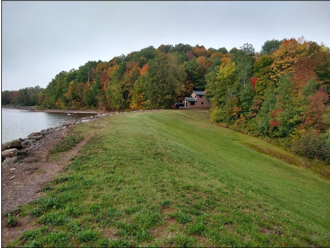
Figure 3.10.1-2 View of Gile Dam Looking West
