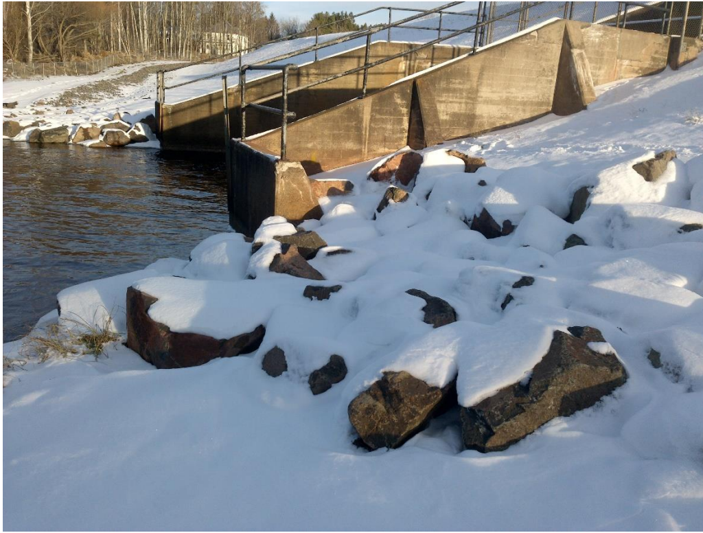
Figure 3.3.1.4-2 Completed Erosion Mitigation
